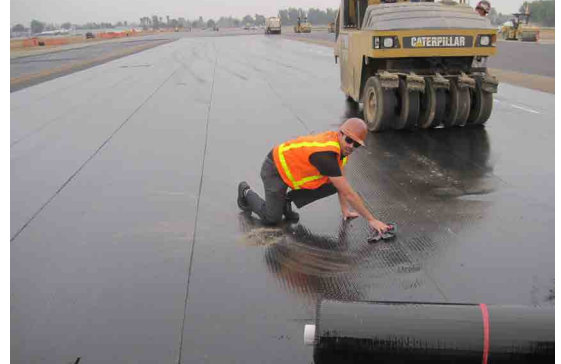
Pic. 3: ADFORS GlasGrid TF installation and rubber roller adhesive backing activation
