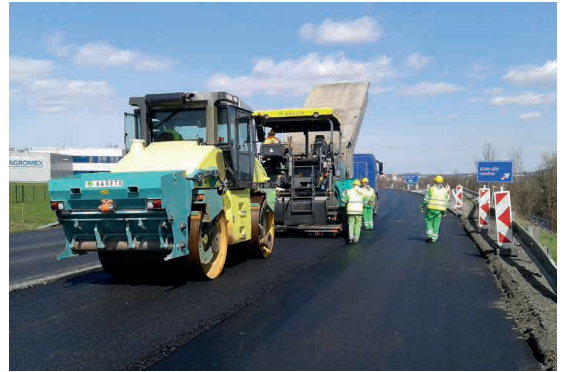
Pic. 9: Pave Overlay
