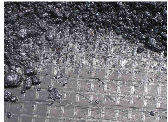
Pic. 7: Film activation by HMA application over ADFORS GlasGrid TF
