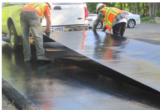
Pic. 2: ADFORS GlasGrid TF installation
