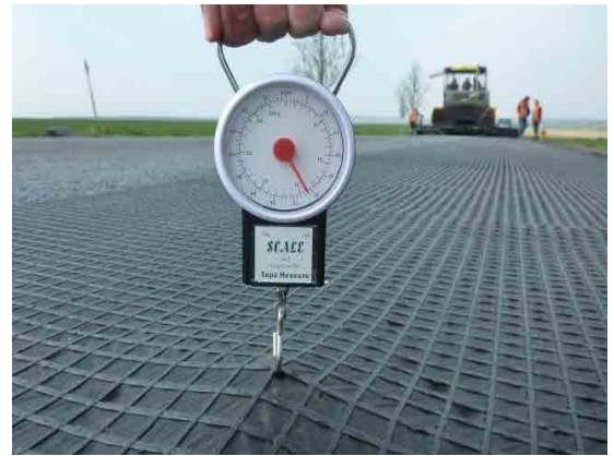
Pic. 6: Adhesion pull out test
