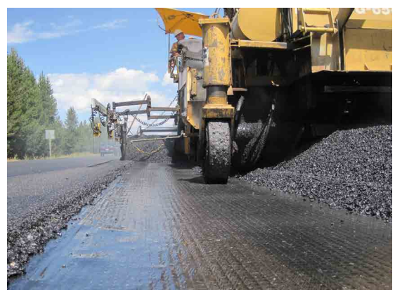
Pic. 8: HMA application over ADFORS GlasGrid TF
